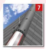
7. Loosely insert the long ratchet clip and two short ratchet clips respectively into the middle and side slots on the union. Lay the ridge tile on the ridge roll, starting at the gable end or hip abutment, and slide the next ridge tile into the open end of the ridge union and press all three clips firmly in place. Secure the union with the screws provided, through the long ratchet clip.
