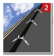
2. Place the ridge batten brackets across the apex of the roof, and nail to the rafters on both sides of the roof, using the nails provided, which can be fixed at 450mmm & 600mm centres. Install the top tiling batten as normal, leaving a 10mm gap before the ridge batten.
