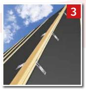
3. Place the first ridge batten in the batten bracket, and nail through the holes provided in the flange. Build up the ridge batten to the required height by adding one or two more battens, nailing each to the previous batten to ensure it is adequately secured in place.
